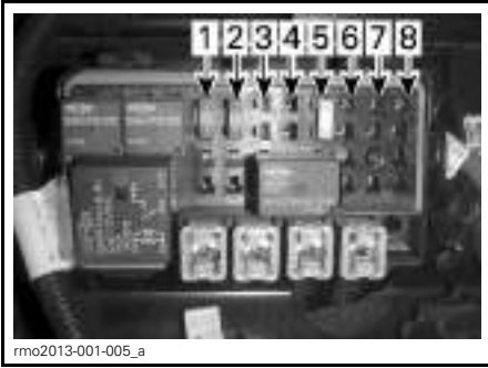
FUSES - RIGHT FUSE BOX
