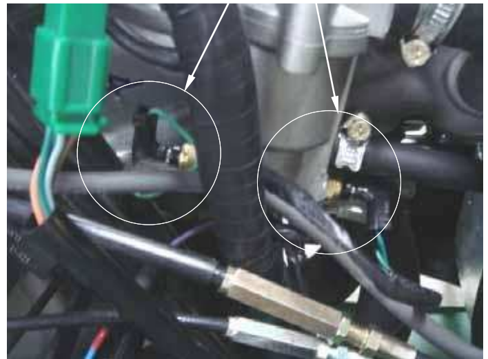
Water temperature sensor
